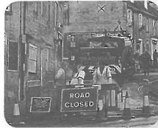
5 Repairs to streets and freeways. (4, 4)
